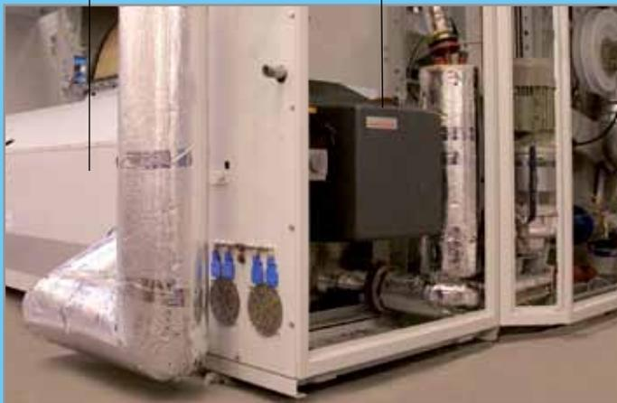
Integrated gas-fired burner and heat exchanger
