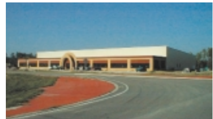
IPSO USA Plant in Panama City (Florida)
